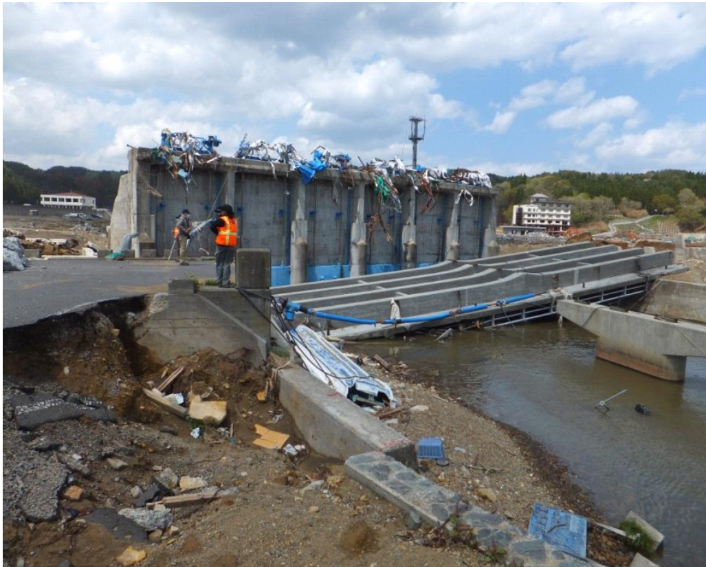
Figure V.4. Field survey of Iwate Prefecture Japan. Georeferenced Photo label is: DSCF0248_5-13-11_Taro Fishing Port_Bridge Deck System Turned Upside Down off Piers Adjacent to Canal Control Structure_RMN.JPG.
